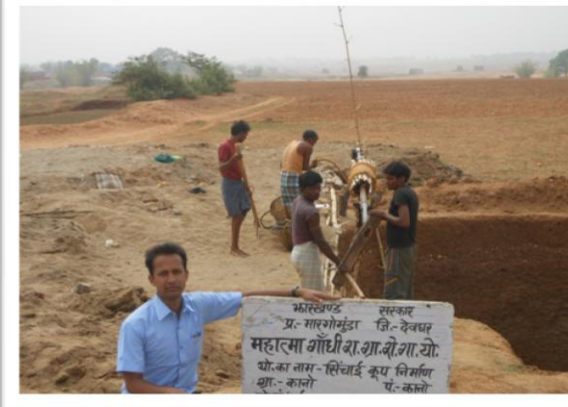
Photo 3 : Well being Constructed under MNREGA
